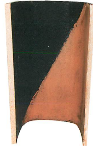
Completely restored flue tile
