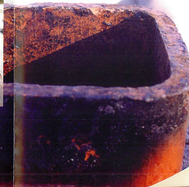
Removal of modified glaze by chimney sweeping
